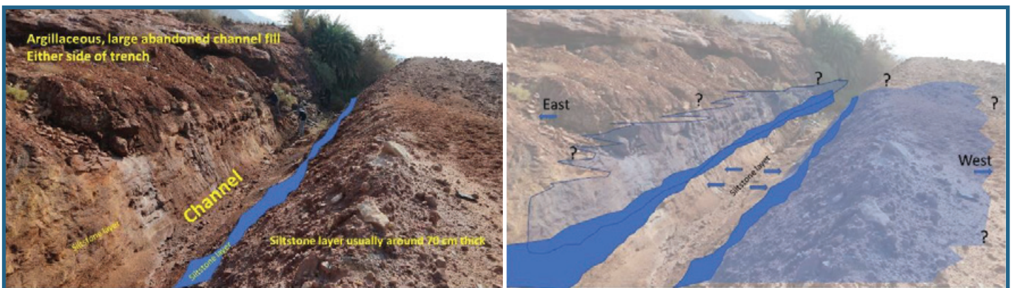
Fig. 5. Large abandoned channel fill exposed in a trench related to a new roadcut
