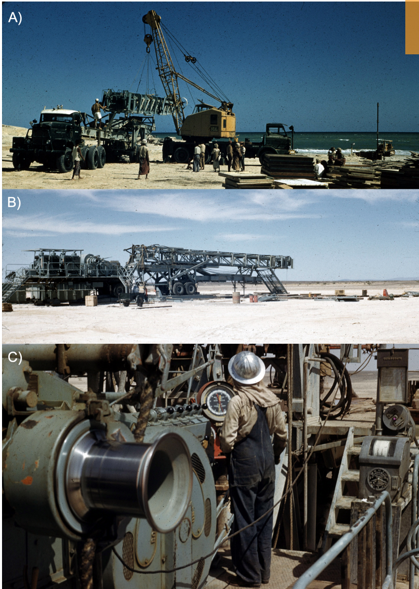
Fig. 9) Woodfield Rambler mobile rig A) being assembled on the beach in Duqm, B) rigging-up on the Afar location and C) drilling Afar - 1(Photo credits- G. Laurance). This rig, handed over to Shell/PDO, would go on to discover oil at Yibal (1962), Natih (1963) and Fahud (1964).
