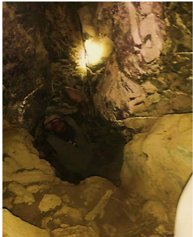
Image 9. Vertical shaft of about 5 m height, connecting multiple tunnel levels.
