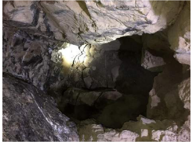
Image 8. Manually excavated 2x2m mining chamber.
